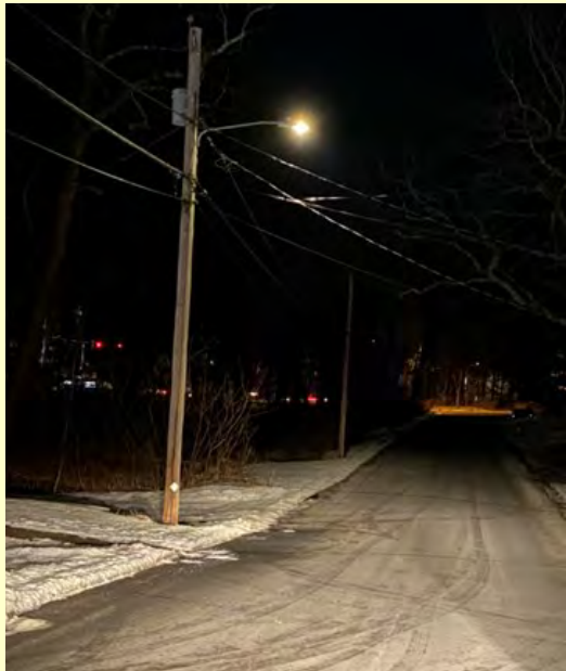
LED Streetlight comparison photos taken on Sibley Street in December 2019. Note the difference in color and reduced glare.
